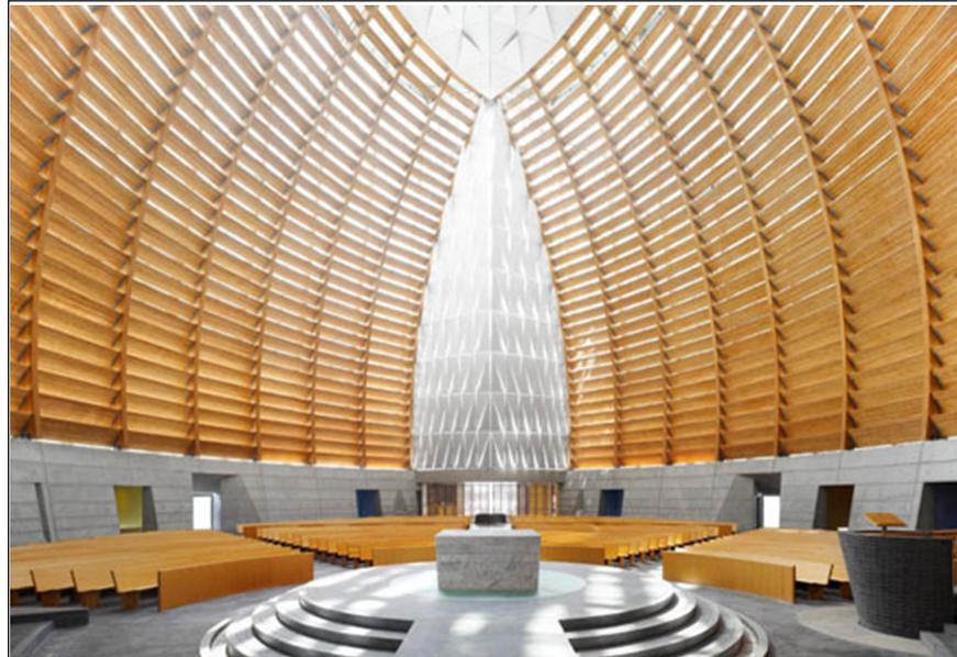
The skylight focuses light onto the center altar, allows views of the sky, and is also part of the unique passive cooling system. The system uses natural convection to cool air as it rises up through floor vents and out through openings in the oculus.
